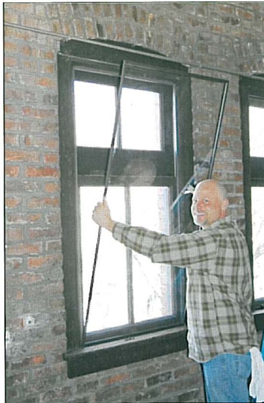
Photo by Julie Stinson [enlarge] Jack Stinson fits a storm window inside the old Fire Station 18 in Ballard.
